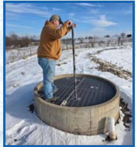
RRWA's Wastewater Superintendent, Richard Brooke, at a lagoon discharge structure.
