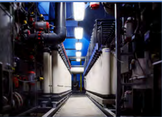
Keokuk uses ultrafiltration membranes to treat water for RRWA.
