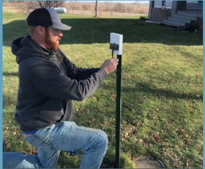
RRWA employee installs smart meter antenna
