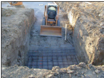
Effluent Pipe Channel Footing
