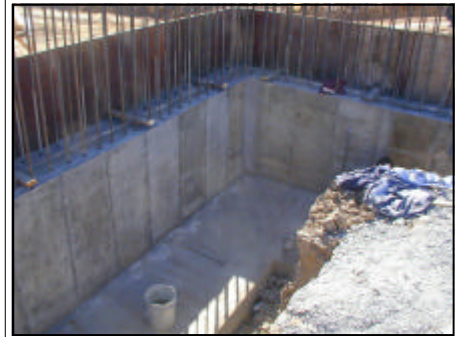
Finished Five Foot Wall
